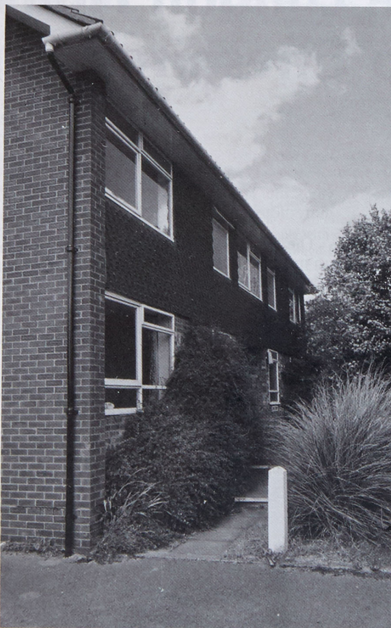
The block of flats at Farnham, Surrey, to be adapted to provide accommodation for mentally handicapped adults.
